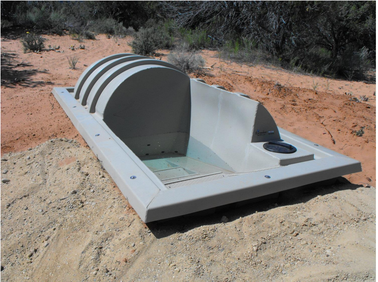
1000-gallon guzzler provided by Rainmaker Wildlife https://www.rainmakerwildlife.com/products/dome-top-500
